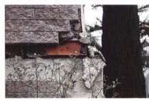
Many buildings with inadequate shear resistance at their base were knocked off their foundations.
