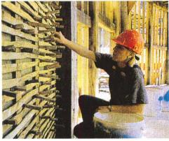
INSTALLATION OF TEMPORARY T-PEGS TO HOLD FIREBOARD IN PLACE DURING THE TUCK-POINTING OF THE PLASTER BEHIND THE OAK LATHS.
