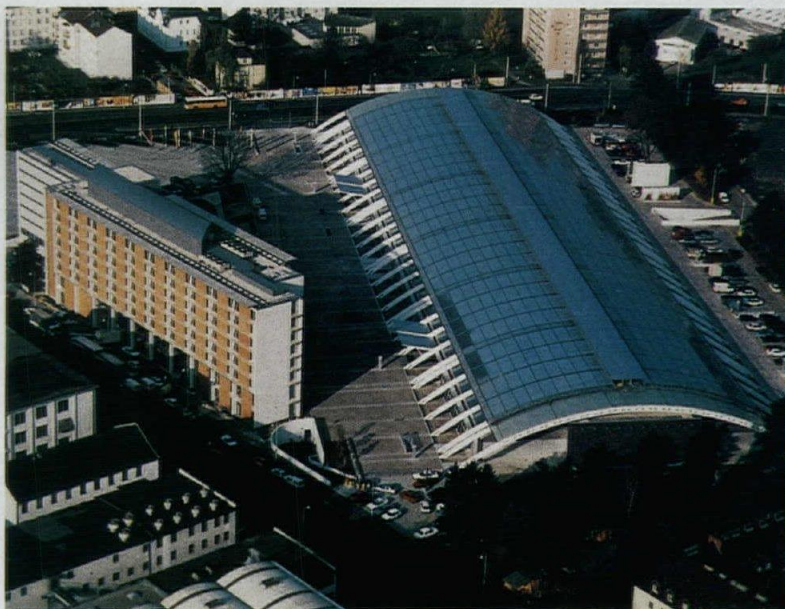
DESIGN CENTER (ABOVE), DETAIL OF ROOF PANEL (LEFT)
