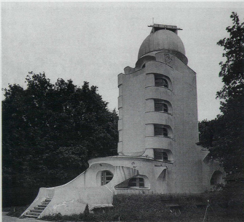
VIEW OF TOWER FROM NORTHWEST, circa 1983
