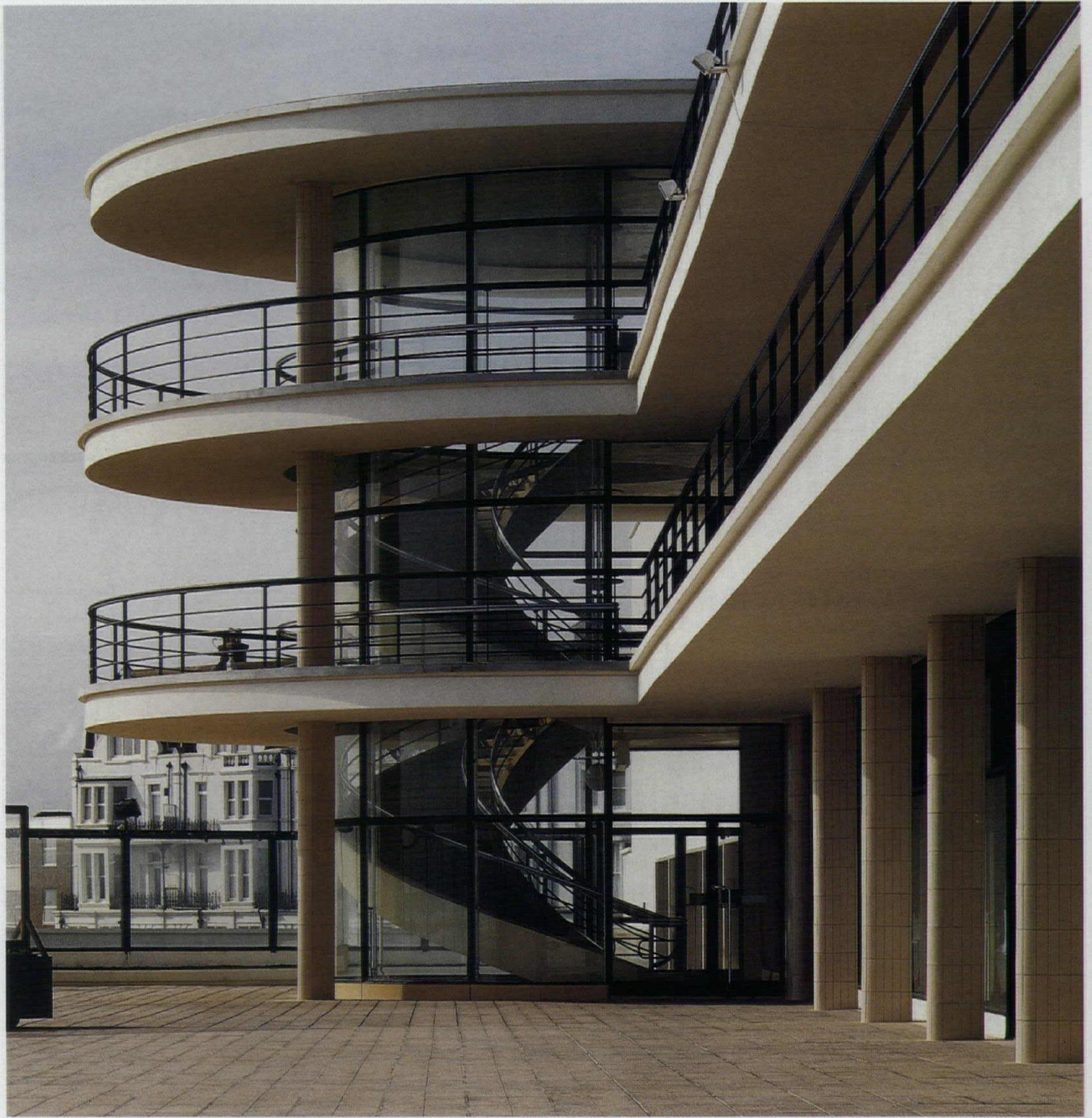
RECONSTRUCTED BALCONIES AND TERRACE ON SOUTH SIDE
