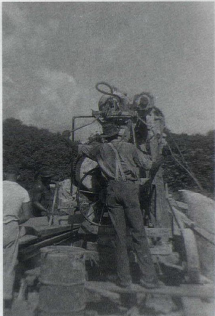
TEXTILE CONCRETE BLOCKS BEING MIXED ON SITE, circa 1940s
