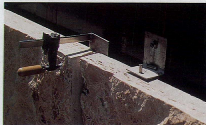
DRY-HUNG STONE MOUNTED WITH BRACKETS
