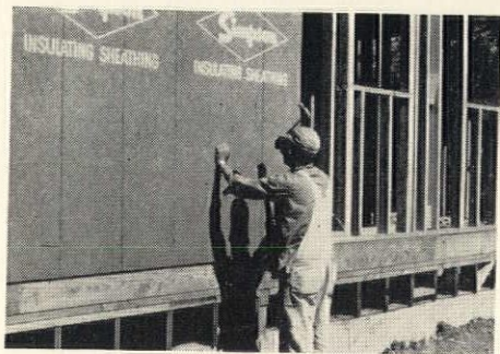
Sheathing is pre-treated for protection against termites, rot, and mildew.
