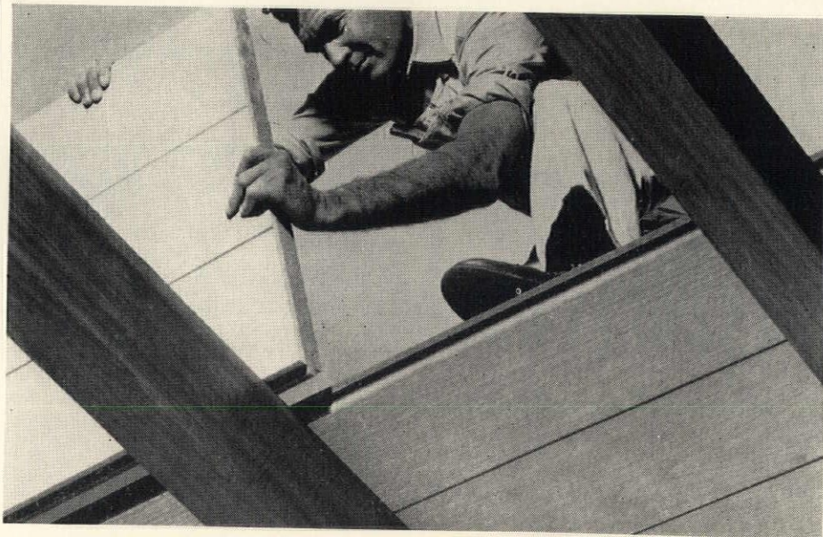
Insulating roof deck may be used in exposed beam construction.
