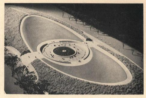
A reinforced-concrete pavilion within a ring of trees and atop a man-made hillock. Eight beams and column elements cantilever in two directions to create a feeling of strength and tension. A precast concrete "lens" is supported at roof center over a larger-than-life-size bust of Roosevelt. Beam separations act as viewing slits toward the other three memorials. Architect: Tasso Katselas; Structural Engineer: Gensert, Williams & Associates.
