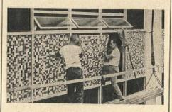
and gives installation details. The tile is set with weatherproof, flexible grout, and is frostproof. An organic adhesive securely bonds the tile to the panel core. Sandwich core is composed of asbestos-cement board bonded to rigid insulating board. Maul Macotta Corporation, 1640 E. Hancock Ave., Detroit 7, Mich.
