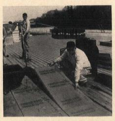
several 11/2"-thick blocks of Foamglas between two layers of laminated kraft paper, with a special asphalt for adhesive. Laminating paper is recessed 1/8" from the edge of the board to permit tightly butted joints that can be sealed with roofing bitumen. Availability of the insulation material in board form speeds installation time and cuts labor for roof insulation applications. Boards are 24" x 48", weigh about 10 lbs. Pittsburgh Corning Corp., 1 Gateway Center, Pittsburgh 22, Pa.
