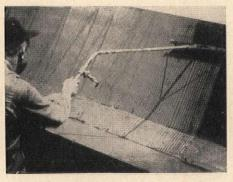
tional spraying equipment, employs two compounds: F/A 400, which is based on neoprene and serves as a primer base coat, and F/A 600, based on Hypalon and providing weather-resistance and color for the surface. Basic color is white, but coating may be pigmented with other colors on request. Thickness recommended is 20 dry mils, producing a surface membrane which will weigh, in most cases, less than 20 lbs per 100 sq ft. Armstrong Cork Co., Lancaster, Pa.
