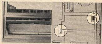
All projected and hopper style windows are weatherstripped with Schlegel deep woven pile to insure a positive seal.
