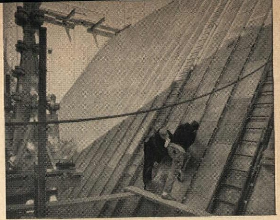
New sections of Washington Cathedral being roofed with lead.
