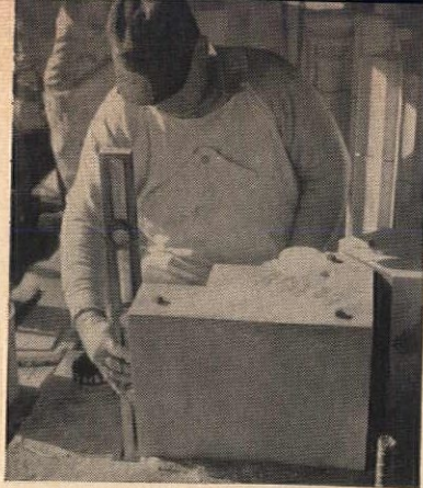
All stone in Washington Cathedral is set on lead pressure-relieving buttons in the joints.
