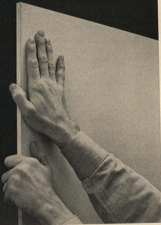
5. Take wallboard. (Forget the vapor barrier.)
