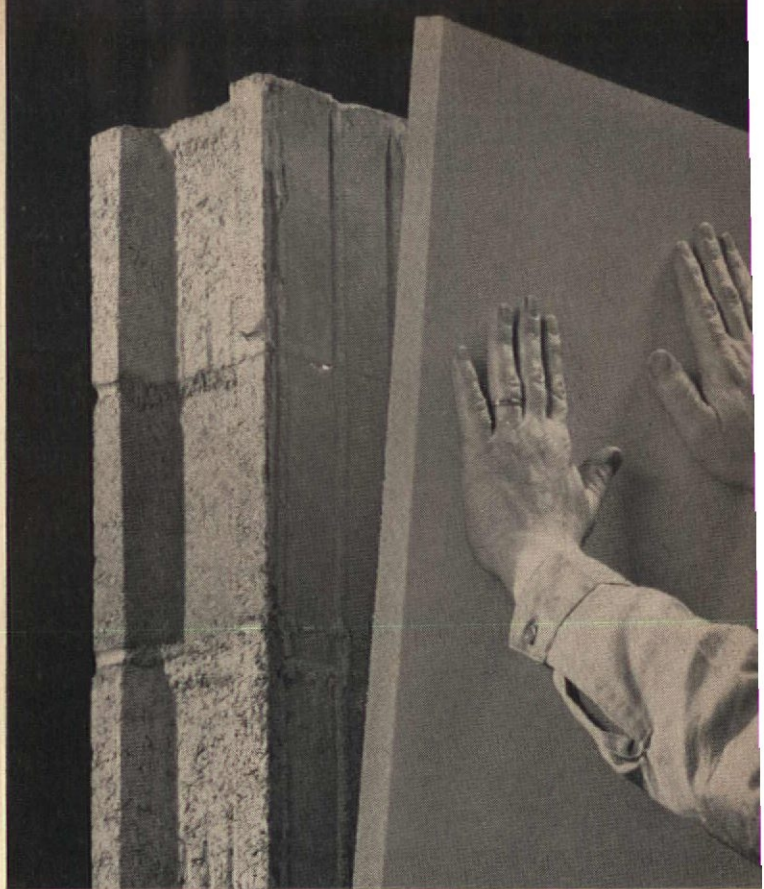
4. Styrofoam FR is pressed into place.
