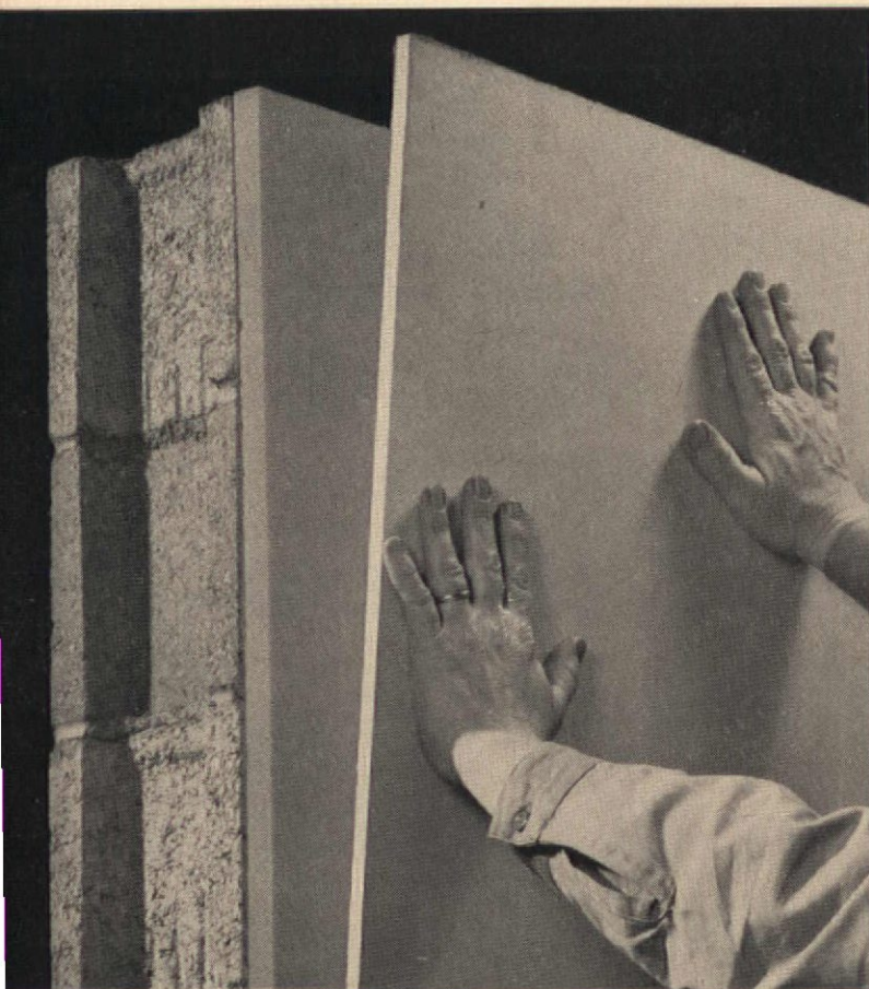
7. Wallboard goes up. Finished wall (8-in. cinder block, 1-in. Styrofoam FR) has U factor of 0.14.
