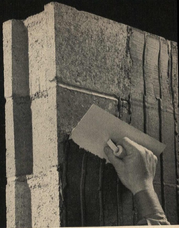
2. Start with Styrotac® bonding adhesive.
