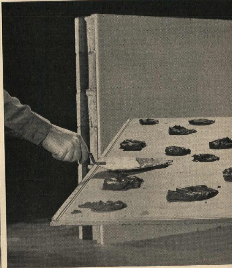
6. Styrotac goes on.
