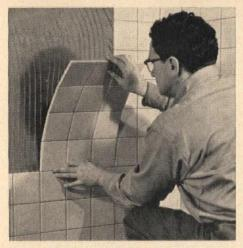
Up goes BETTER-BOND, 12 tiles at a time, with perfect joint alignment and positive bond with setting bed.
