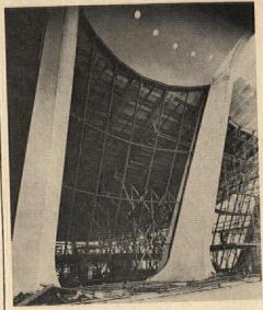
columns in the terminal is approximately 40' wide by 50' high. Neoprene gaskets seal the joints between the mullions and the ½" plate glass and the steel framework. Revere Copper & Brass, Inc., 230 Park Ave., New York 17, N.Y.
