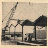
New 8" x 16" Hi-Stress units are fully prestressed slabs ( $f_{\rm si}$  175,000 psi) cast in steel forms, with stress-relieved strands tensioned before concrete is poured. Appearance is similar to standard Flexicore slabs which use pretensioned intermediate grade steel bars.
