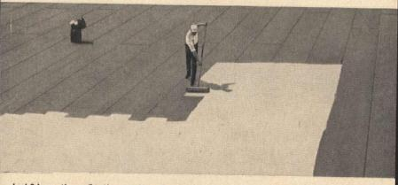
Last-O-Lume, the reflective surface finish, is an elastomer-based coating, formulated for compatibility with all Last-O-Roof membranes and adhesives. It's available in durable aluminum, white and metallic pastel colors to harmonize with any building design. The highly reflective surface will aid in lowering roof and interior temperatures.
