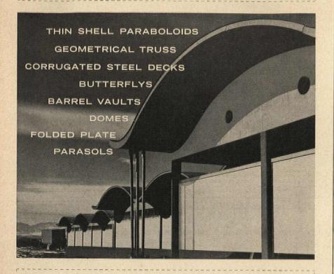
Permalite insulating concrete, with 'k' factors from 0.77 to 0.51, is easily applied to any shape roof deck with standard equipment. Weighs only 3½ to 6½ lbs/sq. ft., 2" thick, with compressive strengths to 500 psi. Permanent. Rot-proof. Fire-proof.
