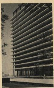
would probably look even more mechanical than it is. What personality it has stems from wrap-around horizontal exterior concrete canopies, cantilevered 15' beyond the exterior steel columns. These canopies, of course, serve as sunscreens, lightening the airconditioning load. The building's 880,000 sq ft gross floor area is heated by bootstrap heating: heat from the lighting fixtures is captured and circulated.
