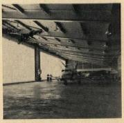
Vinyl-nylon sandwich doors let light into airplane hangars, are said to be secure in winds up to 80 knots and unaffected by extreme temperatures. Electric motors roll 90' x 25' doors up or down in two minutes. Quiet operation, freedom from jamming due to ground heave, small storage space, and economy are said to be some of the advantages. Shown is installation at Cincinnati Lunken Air Transportation Center (doors closed). R.L. Kuss & Co., Findlay, Ohio.
