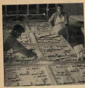
resin for church window-wall panels. Cast glass (approximately 1" thick) is chipped or faceted on interior face to disperse light passing through window. Set in modular steel frames, the glass and epoxy binding are reinforced with steel rods. Conrad Schmitt Studios Inc., 1325 S. 43 St., Milwaukee, Wis. 53214.
