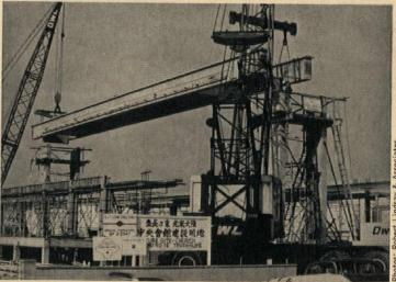
LOS ANGELES, CALIF. Using the traditional form of the Japanese temple, but substituting two precast, post-tensioned concrete beams for wooden roof beams, the firm of Kajima International, Inc., has fashioned the Seicho-No-Ie Church
