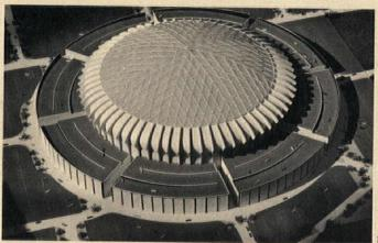
cessfully to attract the Olympic Games.) Movable seats on runners will slide out over the track when it is not in use. Also included in the design is a translucent roof system, supported by an exterior steel grid, in an attempt to avoid the difficulties with vision that the individual skylights in the Houston stadium gave spectators there. The span of the dome will be about 620', and its height above the playing field 270'.
