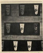
"Flushplate" service outlets for hospitals provide oxygen and suction connections. Sin-
