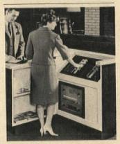
**Control console** for paging and radio sound distribution has AM/FM tuner and 10station switch bank for zone paging. Compact unit is designed for central location such as front desks in motels or hotels. RCA Service Co., Dept. 1614, Bldg. 203-3, Camden, N.J. 08101. *Circle 131, Readers' Service Card*
