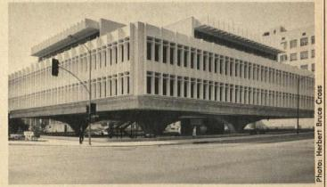
GLENDALE, CALIF. Probably the most striking aspects of the recently completed Municipal Services Building here are the four massively spreading pylons that hold it 21' above street level. At the same time, this stiltlike arrangement merely lets a passer-by see beneath the building to parking lots and streets bevond. The landscaped interior courtyard, which, with its
