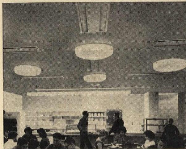
Moduline units in this school cafeteria are separated by incandescent lights, but can still be served by straight-line ductwork.
