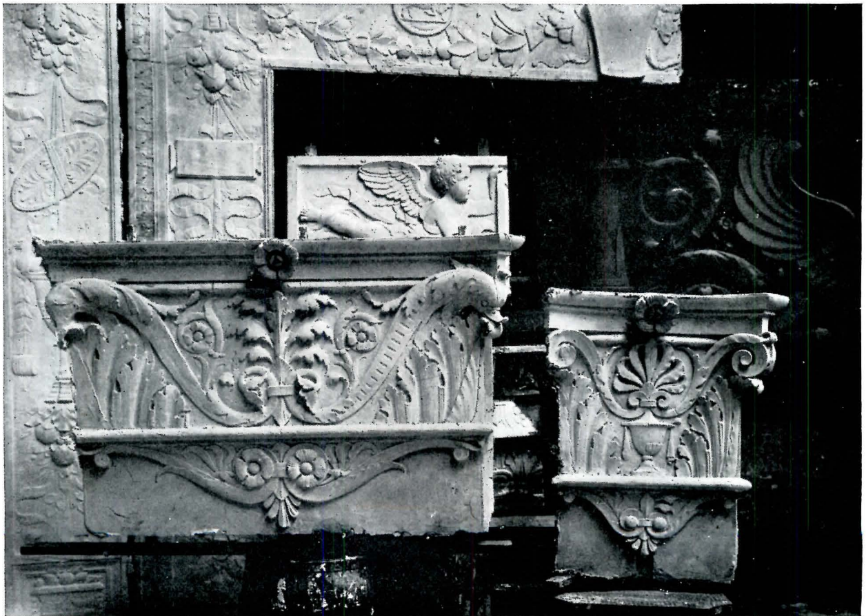
Figure 7. Full-size models of detail, made in sections, with 1\frac{1}{2} in. scale model as guide. They were painted to match color of marble, taken to building, and copied by the stone carvers
