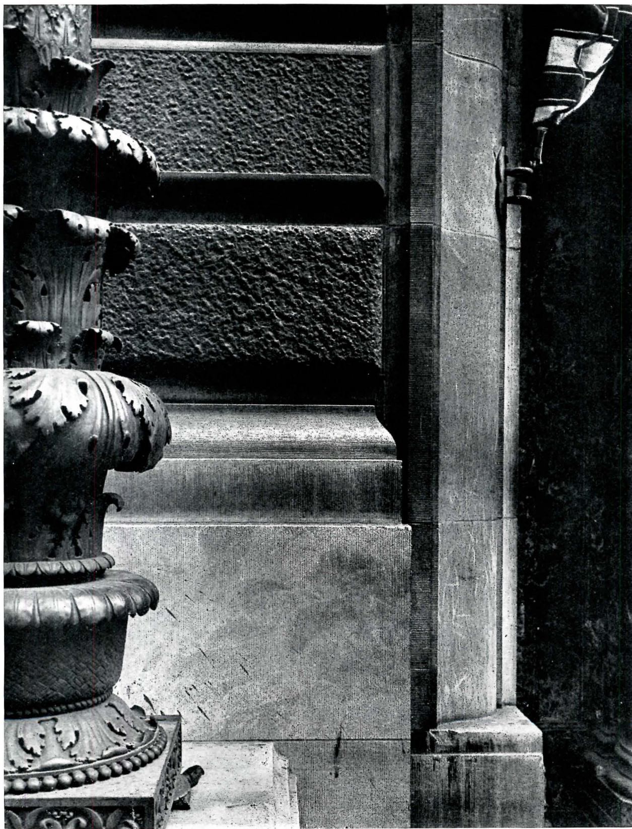
Close-up Photograph Showing Tooling of Stone. Detail of the Union Club, New York City. Designed by Cass Gilbert and John Du'Fais, Architects.
