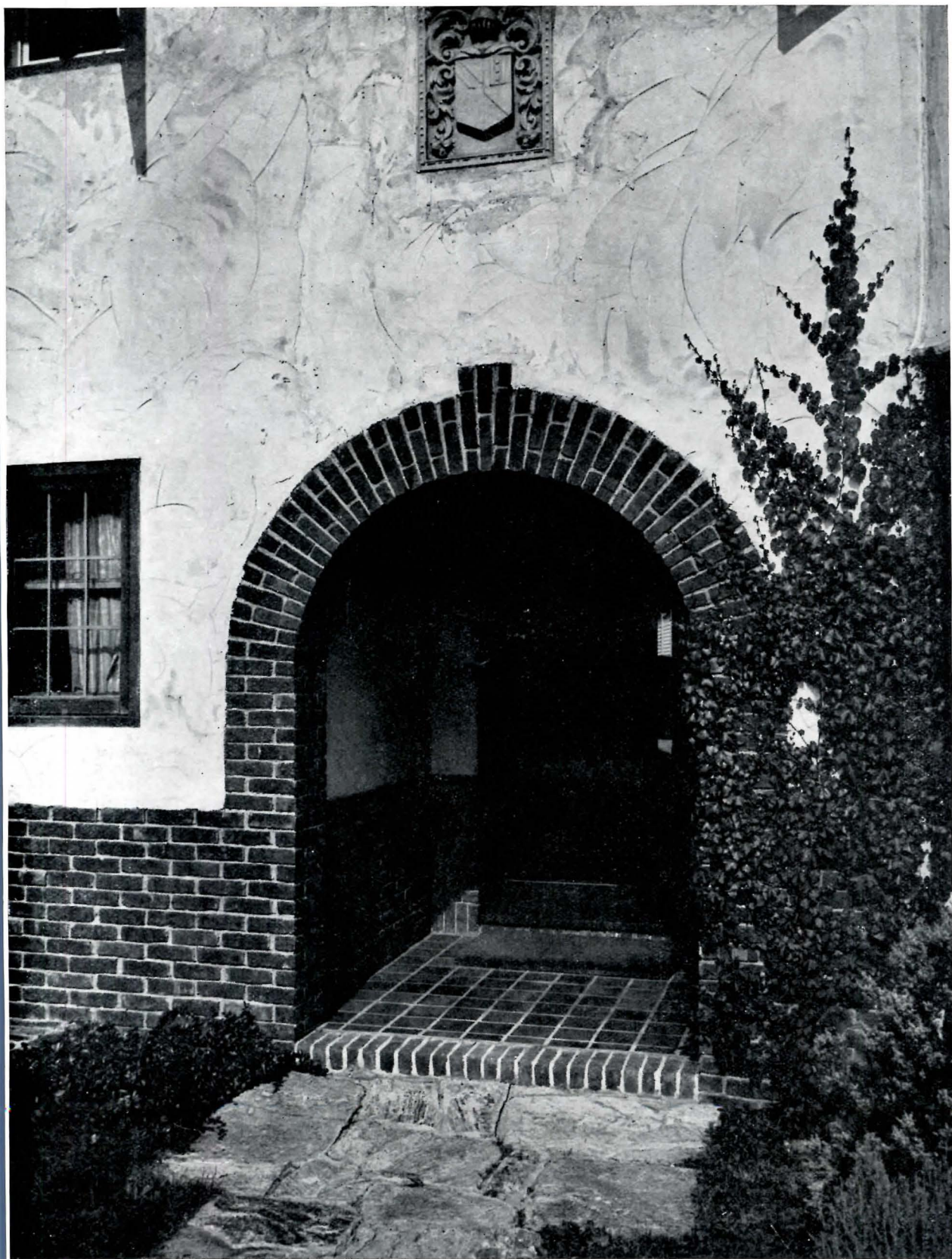
Detail of House for John B. VanHaelen, Esq., Hartsale, N. Y., Frank J. Foster, Architect. An admirable texture in roughly-trowelled stucco.
