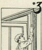
Assemble units, bolt posts, slip on post caps and hang doors.
