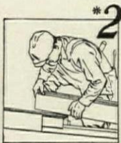
Set base around new enclosure and bolt to floor.
