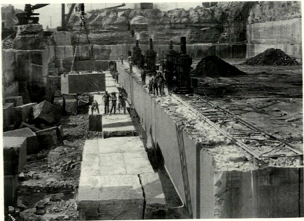
FIGURE 8. BLOCKS NOW READY TO TAKE TO STACKING YARD
