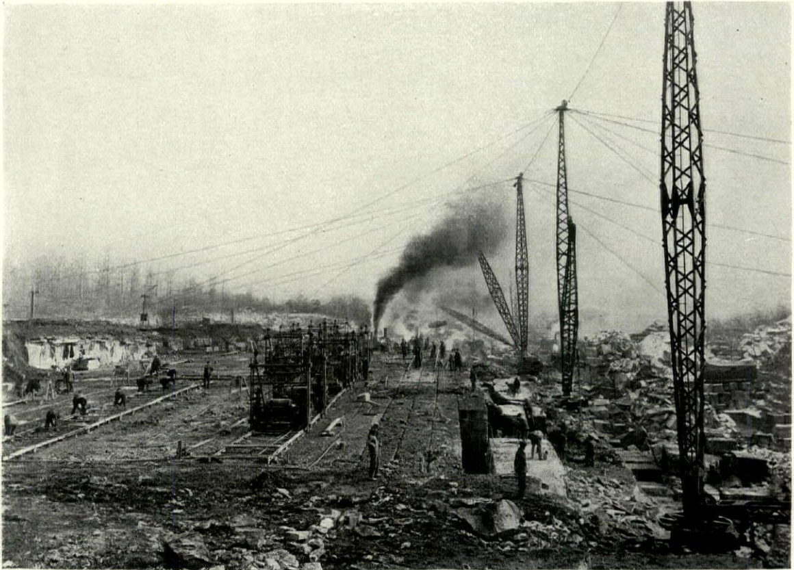
FIGURE 2. CHANNELLING MACHINES IN OPERATION
