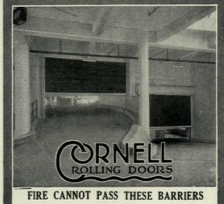
WITH the use of Cornell Automatic Rolling Fire Doors you have absolute protection against the spread of fire within the building. At 150 degrees Fahrenheit the doors automatically roll closed—confining the fire, cutting off draught, safe-guarding property.
