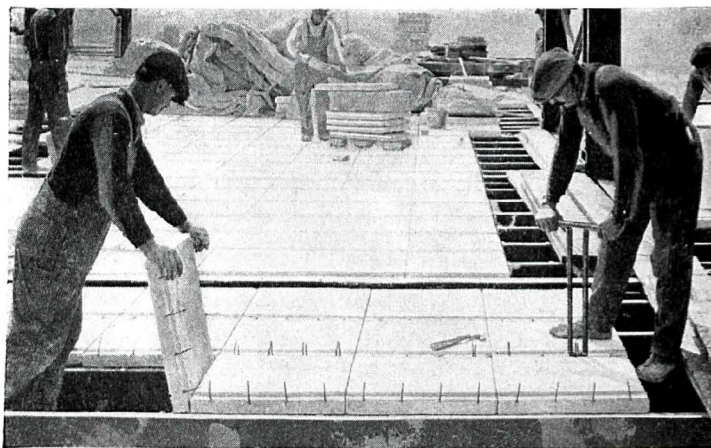
Laying Floor Slabs on top of steel members and tying steel rods together.
