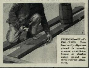
THE Bull Dog Method of anchoring wood floors over concrete saves valuable construction time. No fill to dry—no beveling or shimming—sleepers and finished floor are laid at one time.
