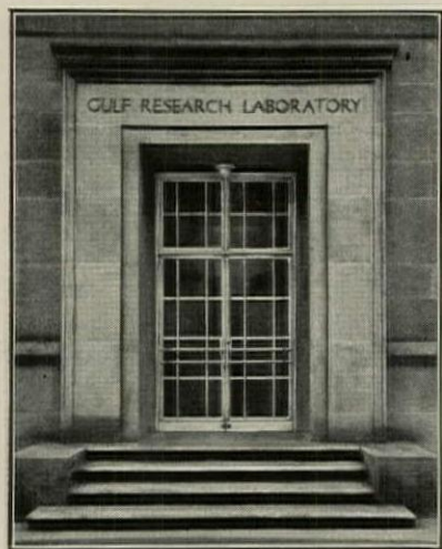
The main entrance doors were fabricated from Alcoa Aluminum and both extruded shapes and plate were used.
