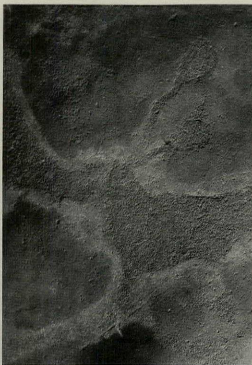
Area of plain concrete floor surface in railroad station, showing effects of sulphuric moisture from overhead track cinders. Sulphuric acid test (Robert W. Hunt laboratories, Test No. 58769) shows Omicron concrete more than six times as resistant as plain concrete, after both immersed 21 days in 1/2% sulphuric solution.
