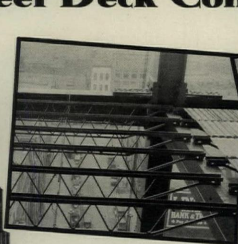
R-G Channel Joists in place ready for Steel Deck fireproofing and bridging forms.
