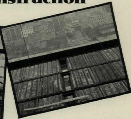
Close-up of bridging beam forms which are integral with and are suspended from steel deck pans for forming solid concrete beams six inches wide at right angles to steel joists.
