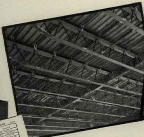
View of under side of R-G Steel Deck Construction after pouring.
