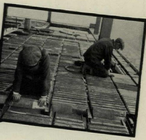
Workmen installing steel deck pans and girder fireproofing forms at 14th floor level.
