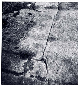
The corrosive action of lactic acid has shortened the life of this milk products plant floor.
