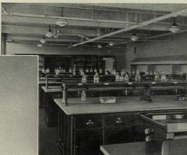
One of the laboratories, showing Duriron drain piping hung from the ceiling.
