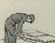
Laying Gypsteel floor slabs
