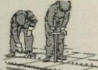
Tying the reinforcement together.
