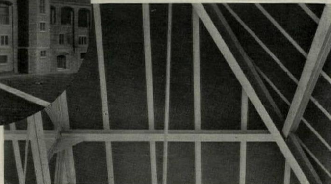
The 6" x 24" trimmings from the full-size sheets of Novoid Corkboard were used to insulate around the dormers.
