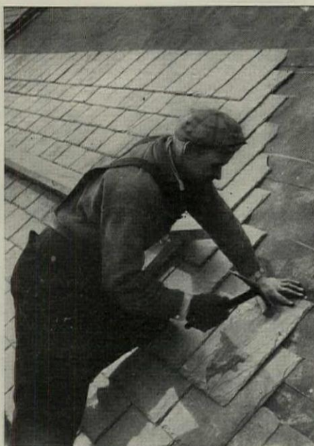
Ebenezer Community Building, Chicago, showing how slate is nailed directly to the roof-deck of Federal Nailing Concrete Slabs. Archt., Andrew E. Norman.
