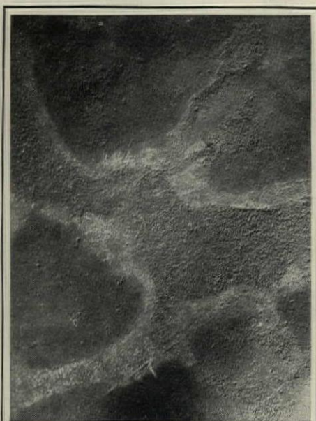
This floor section bore no abrasive wear. The corrosive action of acid-bearing moisture caused the disintegration shown.
