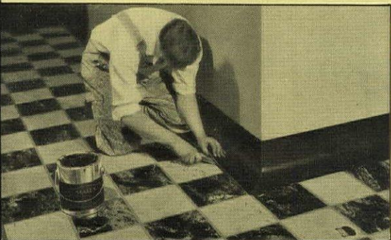
Picture shows mechanic completing the job, spreading linoleum paste under edge of the border and the patterned linoleum used for the floor.
