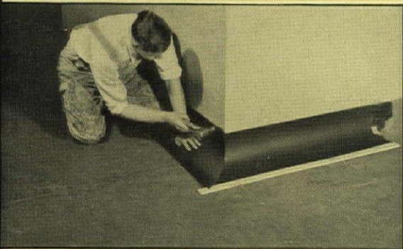
Here we see the mechanic fixing the cove-base and border in place by means of headless brads, placed on 3" centers, 1/4" below top of base.
