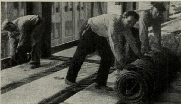
Wire Fabric being laid on floors of Carew Tower
