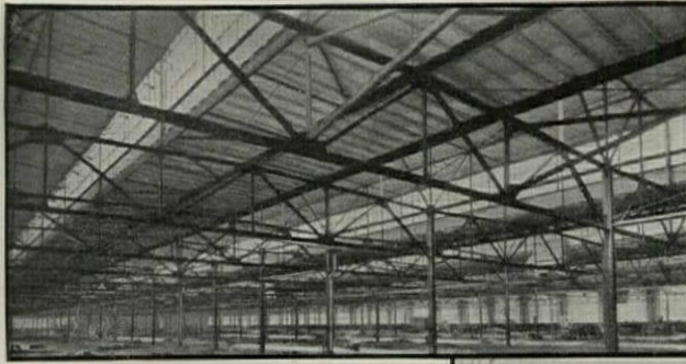
Bendix Aviation Building, South Bend, Indiana. Below—roof deck ready for composition covering . The entire roof of Featherweight slabs was erected in winter—an area of over 300,000 sq. ft. And this expanse represents but half the area of Federal roofs in use by this company!
