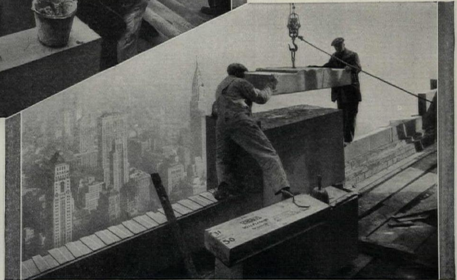
Right: Setting coping stones onto the mortar bed which has been laid over the flashing.
