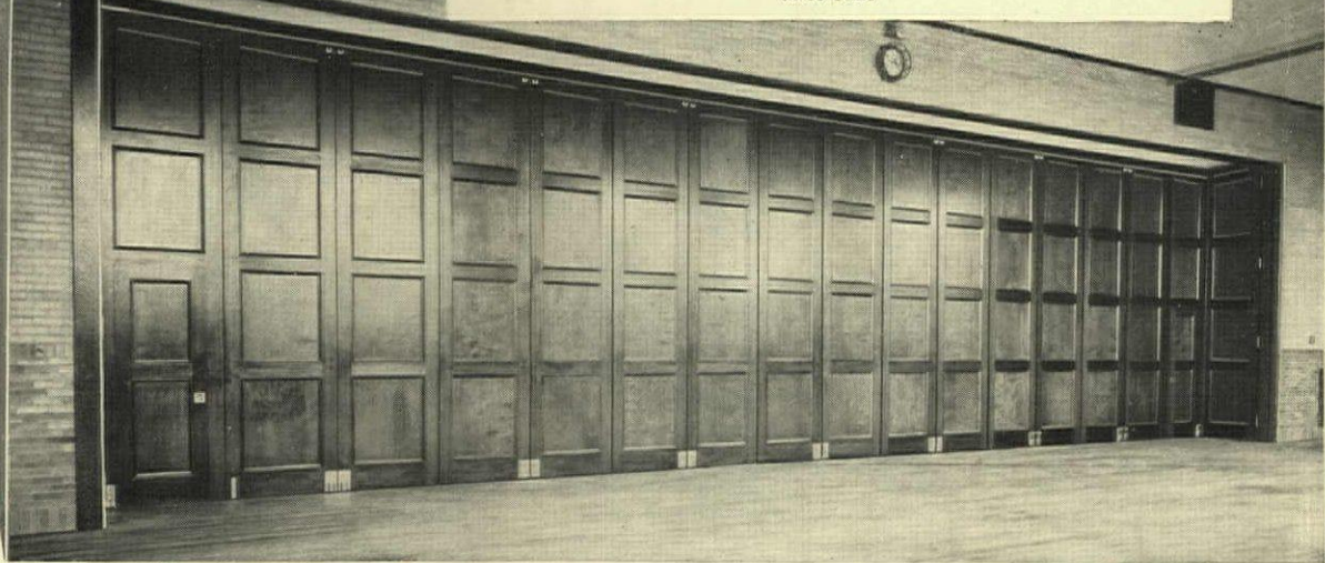
32-door FoldeR-Way installation at Jefferson Junior High School, Jamestown, N. Y. Auditorium and gymnasium are separated by two batteries of 16 doors each, enabling both rooms to be used simultaneously if desired; or providing a stage of three sizes
