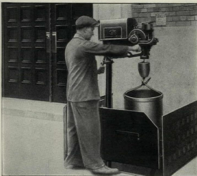
Model E Electric Hoist as used in bank buildings. Note how sidewalk opening is fully protected
