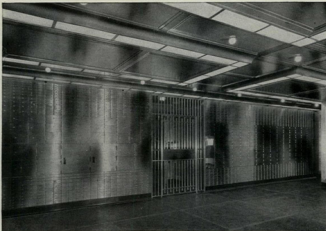
Monel Metal was used for all interior trim of this vault in The Canadian Bank of Commerce, Toronto. Architects: Darling & Pearson, Toronto. Consulting Architects: York & Sawyer, New York. Fabricators: Goldie & McCullough Co., Ltd., Galt, Ont., and J. J. Taylor, Ltd., Toronto.
