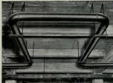
A 6" expansion loop in the Empire State Building, fabricated on the job from 90° Tube-Turns and straight pipe.
