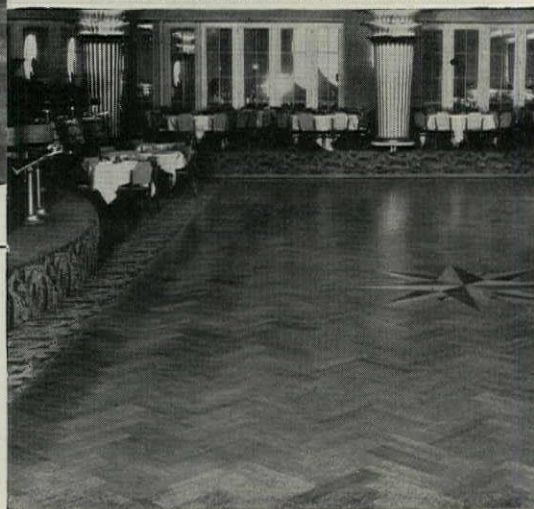
Pavilion Caprice (Night Club); dance floor in mastic blocks of quarter-sawed white oak, herringbone pattern. Note star motif in center panel reproduced in satinwood and teak.
