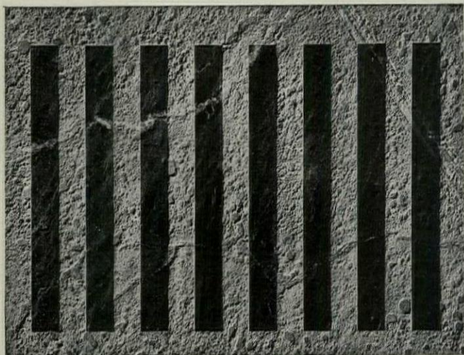
Alberene Stone Spandrel — showing shadow-effects by sand-blasting instead of deep reveals. Stone — one and one-half inches thick.
