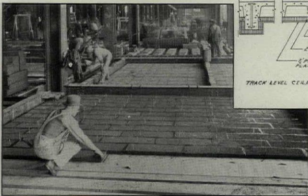
Workmen installing 172,000 board feet of Armstrong's Corkboard over the track level of the Merchandise Mart. Cork serves throughout the building.
