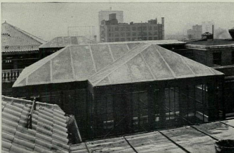
Bellevue Hospital Pavilions, New York City, showing Featherweight Nailing Concrete Insulating Roof Slabs ready for the ornamental covering to be nailed on. Architect: C. B. Meyers.
