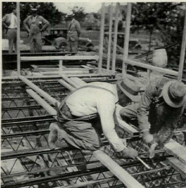
EXPERIMENTAL FERRO ENAMEL RESIDENCE NOW UNDER CONSTRUCTION AT CLEVELAND, OHIO
