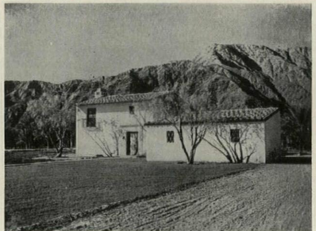
HOUSE BY GORDON B. KAUFMANN, ARCHITECT
