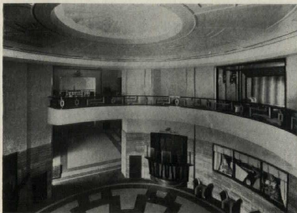
Two views of the main lobby and sala d'aspetto
