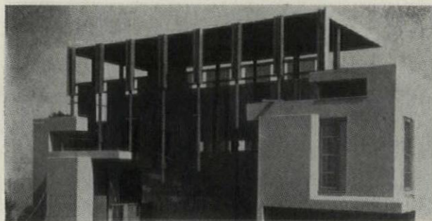
"The House on Tiptoe," by R. M. Schindler Reproduced from "California Arts and Architecture"
