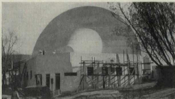
Rear view of the pavilion near completion
