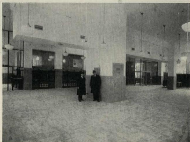
A Robbins Block Flooring Installation
