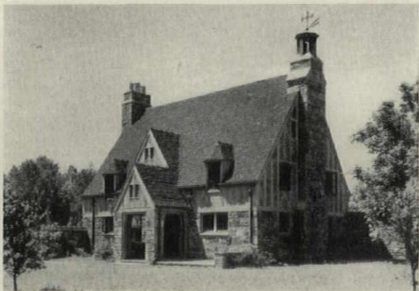
Gate and Lodge of the Acadia National Park. Grosvenor Atterbury and John Almy Tompkins, Architects.
