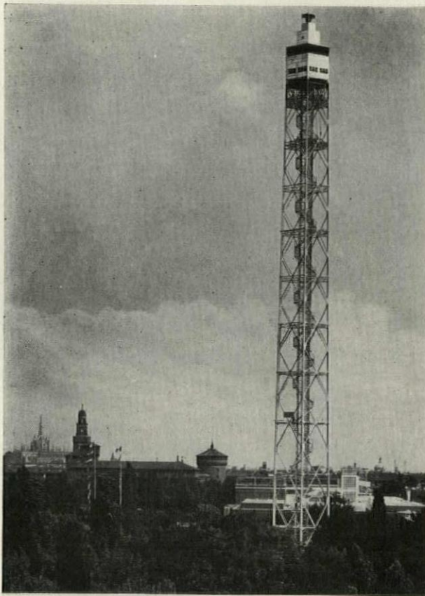
Milan's version of the Eiffel Tower. Ponti points with pride to its construction of tubular steel, its twelve-table restaurant at the top, and to its elevator, the fastest in Europe
