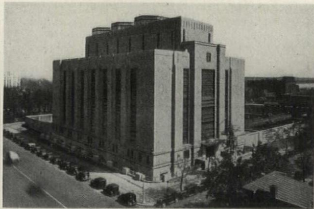
Central Heating Plant, Washington, by Paul P. Cret, Architect From The American Architect
