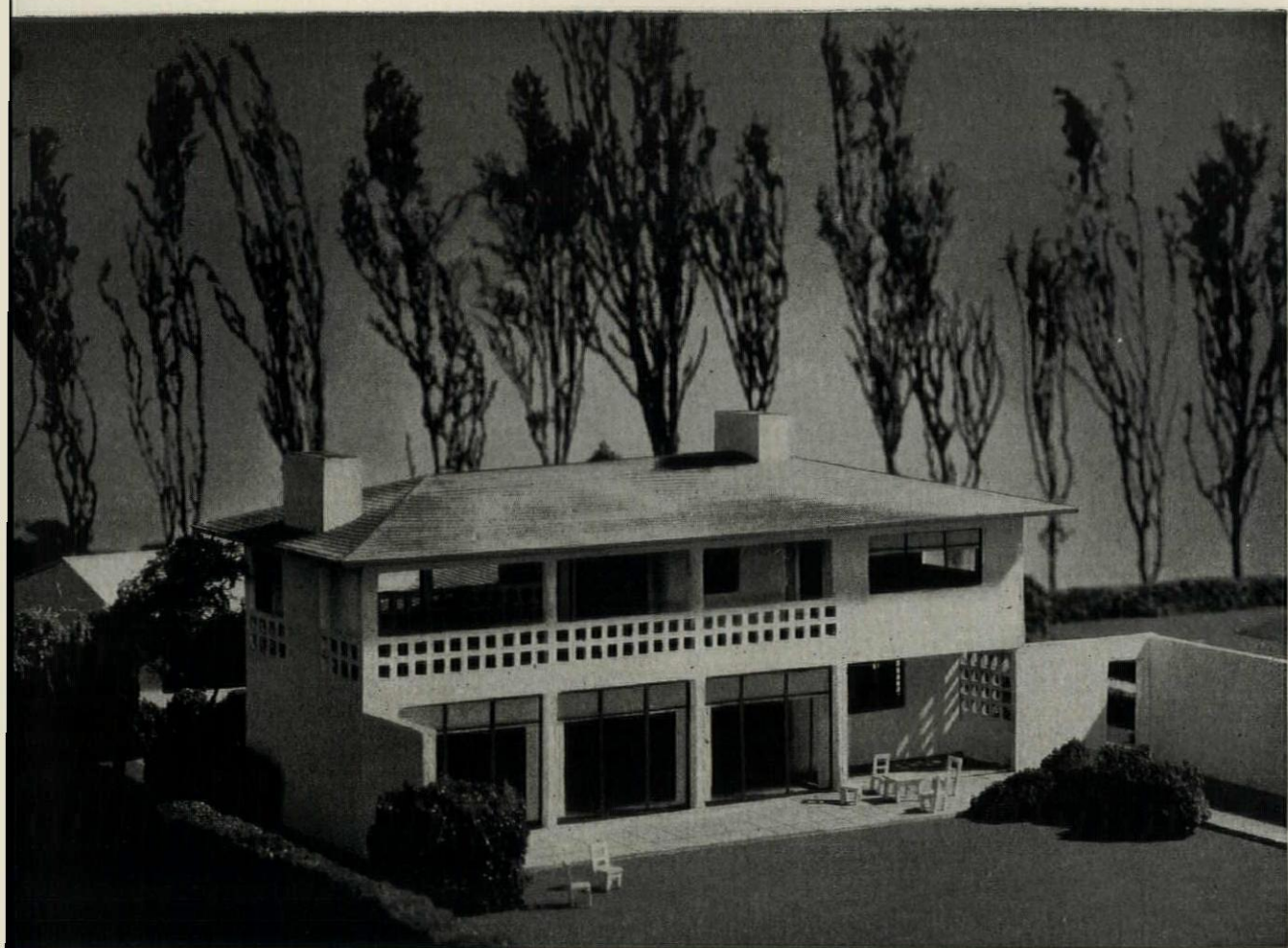
● AIR CONDITIONED HOUSE ( Southern Climate ) that won the Grand Prize ($2,500) in Classes C and D (medium size homes) in the "Home Electric" Architectural Competition, sponsored by the General Electric Company. Architects, Paul Schweikher and Theodore W. Lamb, Chicago. Photograph of small model, made from architects' plans reproduced by courtesy of "House & Garden."
