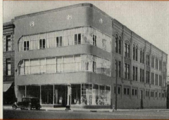
This old-style building was modernized with colored blocks, vitreous-enameling on Toncan Iron Enameling Stock and edged with ENDURO.
