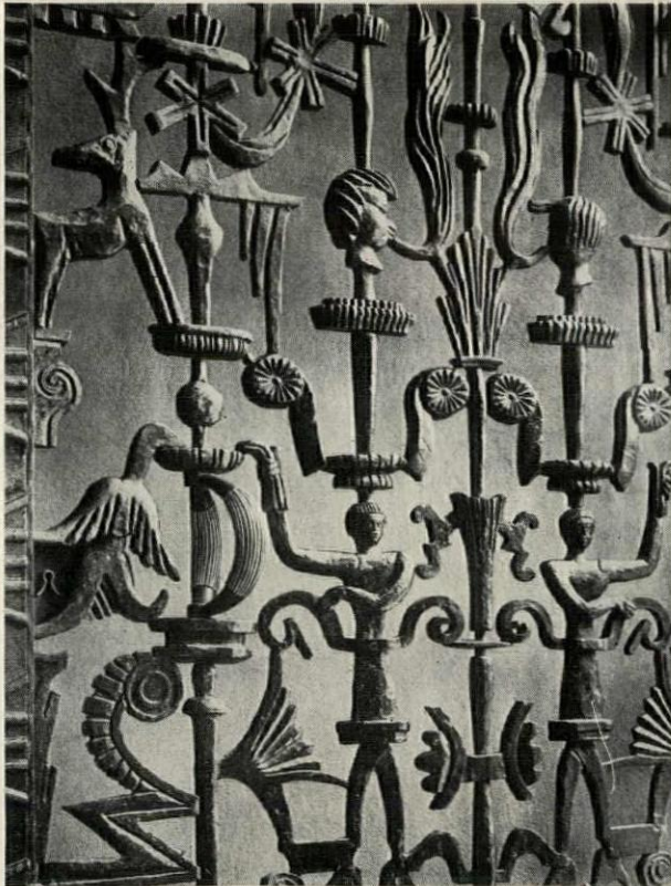
A detail of the main entrance gates showing the rich texture and intricate design. Swedish Match Company Building
