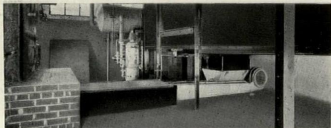
This Iron Fireman boiler room modernization job for Republic Bank Note Co., at Pittsburgh, started paying immediate dividends by cutting their fuel costs 33 1/3%, and reducing firing room labor 65%.
