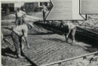
Expanded Metal and Welded Wire Fabric for road reinforcement. It's Wheeling Steel.
