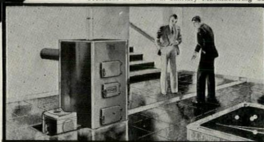
Residential Iron Fireman Coal Flow model that feeds coal direct from bin to fire; for hot water, steam or vapor-vacuum boilers and warm air furnaces.
