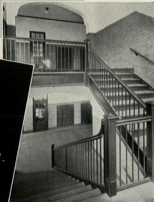
A school stairway installation combining beauty with strength. J & L 12" Lightweight Channels are used as stringers to give the convenience of wide treads with perfect safety.
