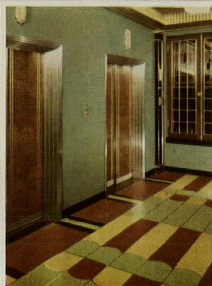
striking floor treatment of Atlas White terrazzo installed in the W. O. W. Insurance Building, Omaha. Architect, Leo A. Daly; Terrazzo Contractors, Nebraska Terrazzo & Mosaic Co., both of Omaha
