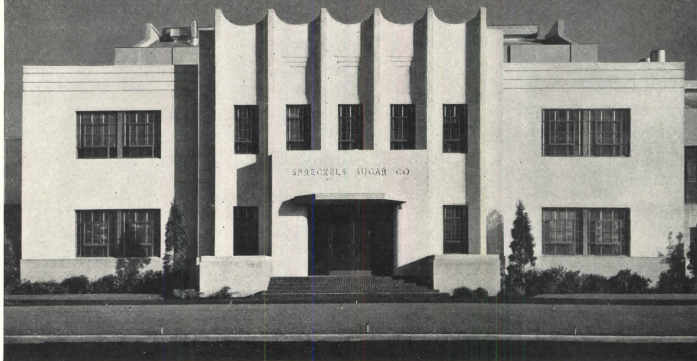
The Spreckels Sugar Company Plant No. 3, near Woodland, California, includes administration building and laboratory, warehouse and five bulk storage bins—all of reinforced concrete with concrete floors. Designed of reinforced concrete with concrete floors. Architect, Harry A. Thomsen, Jr., successor to George W. Kelham; contractor, Dinwiddie Construction Co.—both of San Francisco.
