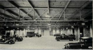
Inside the garage. Note the neat, uniform surface of the PLANK roof-deck, which is laid directly over the steel purlins.
