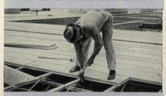
PLANK is a dry job—no mixing, pouring or waiting for materials to set. Can be installed by your own crew.
