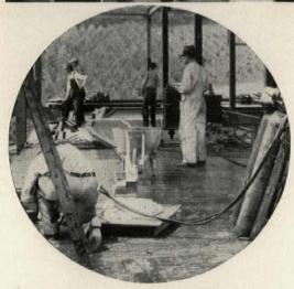
There is no waiting for materials to cure—there is no debris to clean up when you build floors and roofs with Wheeling Long Span Steel Joists. This modern system also saves the cost of extra scaffolding; as exterior masonry work can be done directly from the floor deck.
