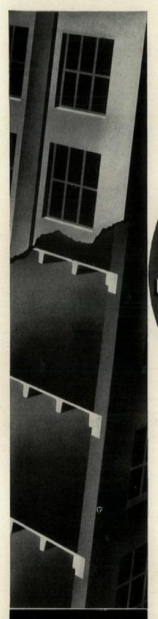
• Substantial reduction of the "dead load" in any structure automatically results in lower construction costs. Concrete Joist Construction definitely reduces "dead load" without sacrifice of permanence, beauty
