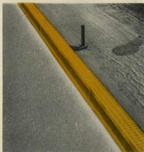
Public Service Co. of N. J., Auto Maintenance Shop, Newark, N. J. Water had been seeping through the fire separation wall. Anaconda Through-Wall Flashing and Anaconda 16 oz. crimped copper counter flashing were installed by L. Himmel & Sons, Newark, N. J., to make the wall leak-proof.
