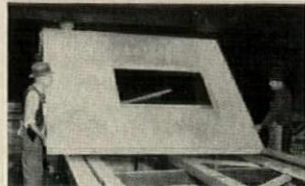
Wall and partition units are framed from working drawings, with doors and windows integral.
