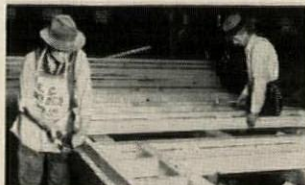
Precision-Built construction starts in the shop—where all lumber is pre-cut.
