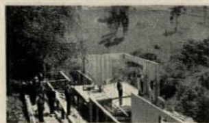
In 2 hours all partitions are up; the job is ready for roofing with pre-cut rafters.
