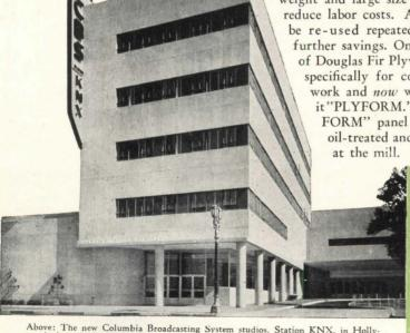
Above: The new Columbia Broadcasting System studios. Station KNX, in Hollywood, designed by William Lescaze, architect; Earl Heitschmidt, associate. William Simpson Construction Co., builders. "Experience has taught me that if exposed concrete is to be the finished surface, best results are obtained with Plywood forms," says Mr. Lescaze. "We are extremely pleased with the results achieved."
