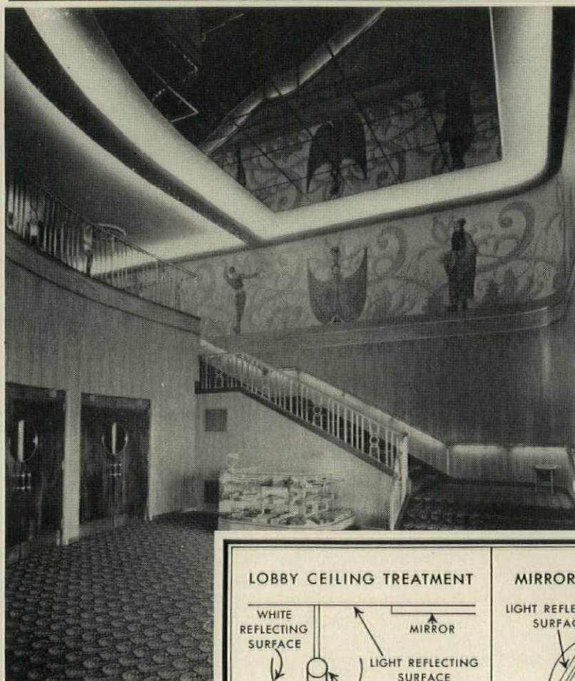
The new Lakewood theatre lobby in Dallas is lighted with daylight fluorescent MAZDA lamps, used in silhouette strip lighting of the mirror ceiling. E. C. Zrenner of the Interstate Circuit, and H. F. Pettigrew, architect, planned this installation.
