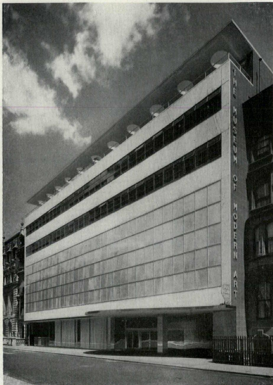
The great thermolux window and pierced, cantilevered slab sheltering the members' terrace on the top floor of the Museum of Modern Art—distinctive notes of the 53rd Street façade—are clearly shown in this photograph taken by Wurts Brothers
