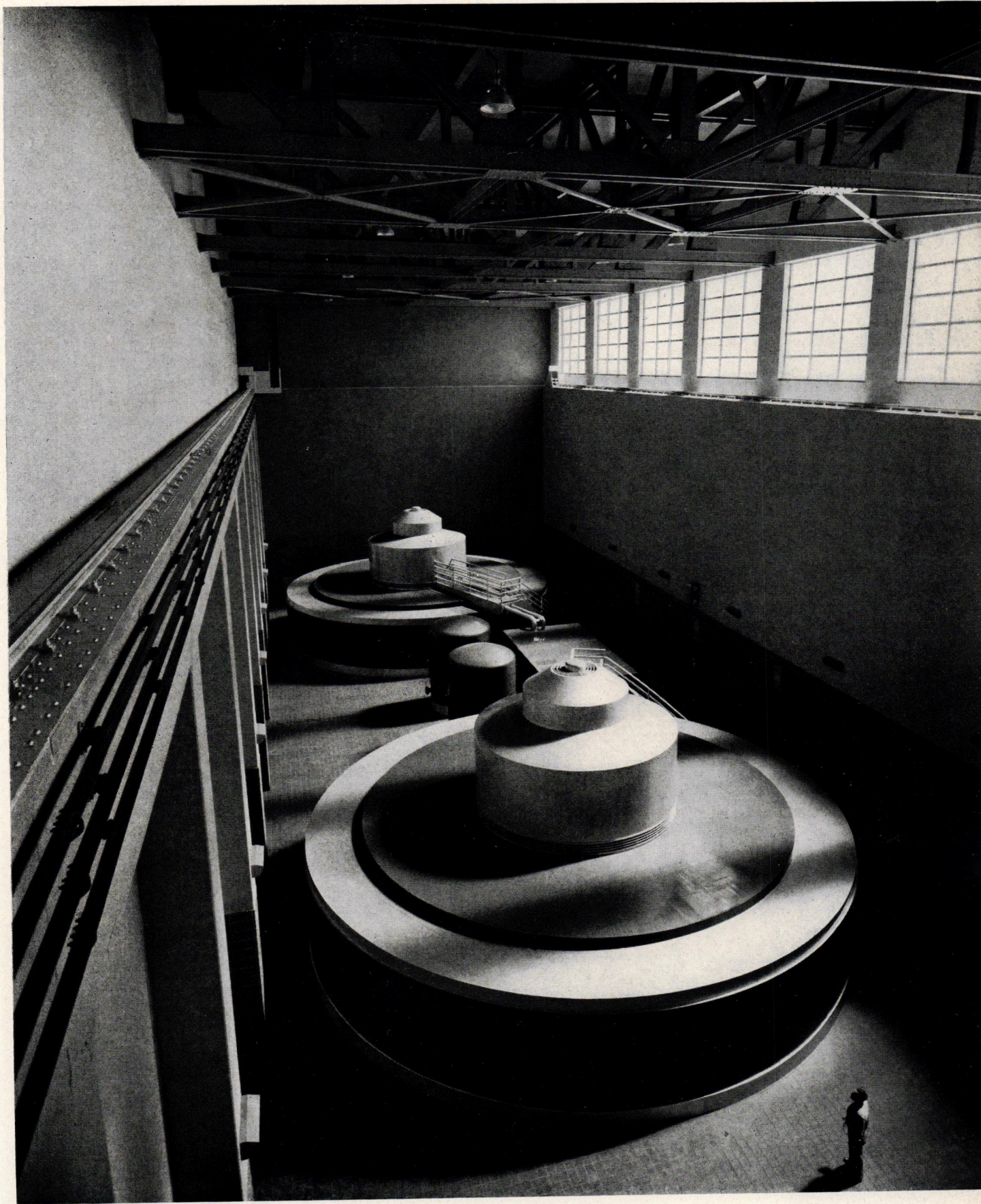
THE GENERATOR ROOM FLOOR AT PICKWICK IS FRENCH GRAY CERAMIC TILE; THE WAINSCOT, EGGSHELL-GLOSS GLAZED TILE OF A GRAY-BLUE-GREEN COLOR. CONCRETE ABOVE WAINSCOT IS PAINTED A LIGHTER SHADE OF THE SAME COLOR TO THE CRANE RAIL LEVEL, THENCE LIGHT SULFUR YELLOW TO THE TOP. TRUSSES AND ROOF PAINTED GRAY, WINDOW PIERS ALUMINUM
