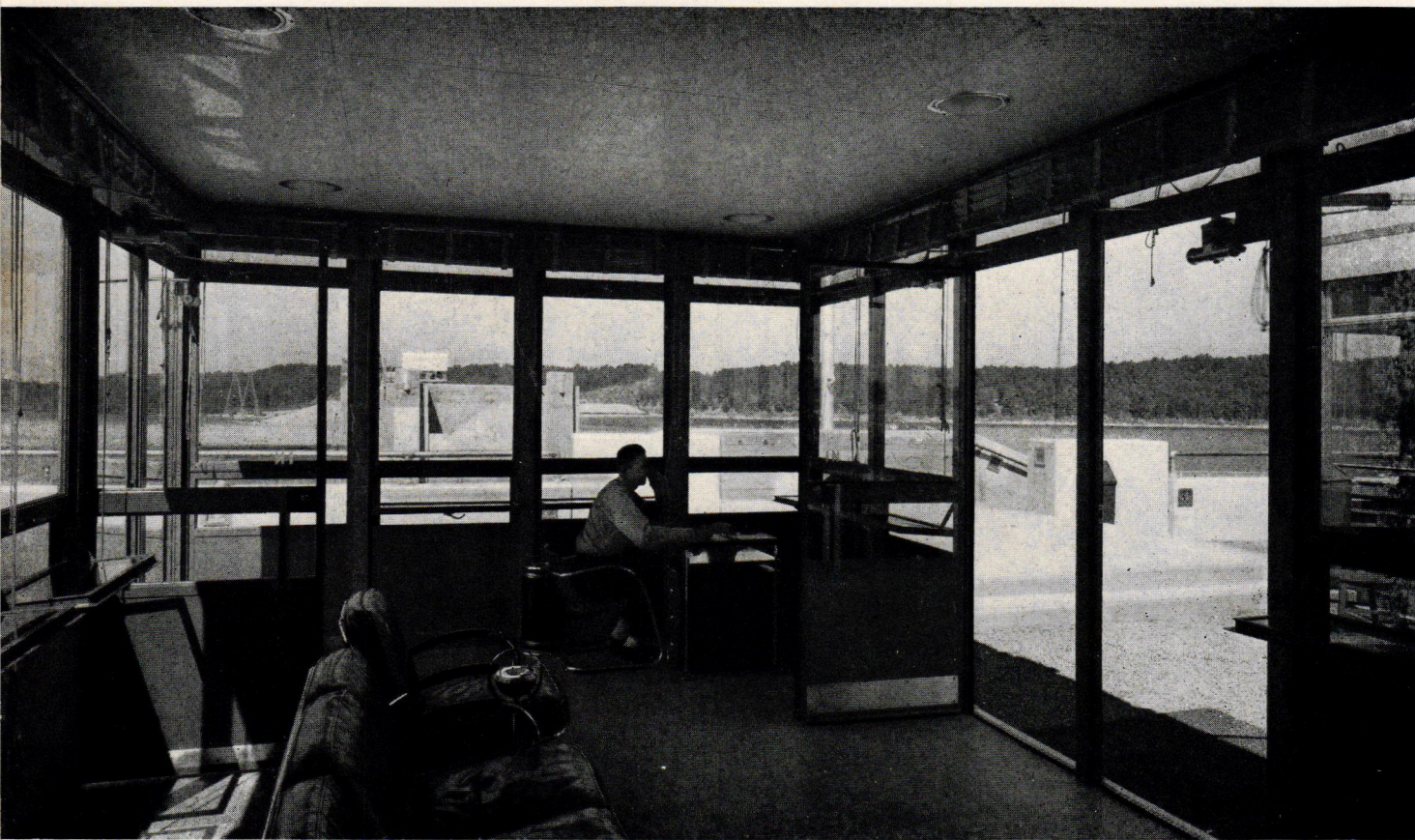
ON THE INTERIOR OF THE PICKWICK LANDING RECEPTION BUILDINGS THE WALLS ARE FINISHED WITH 40" WIDE SHEETS OF 3/16" STEEL-PRESSED, FLEXIBLE, ASBESTOS BOARD OF A MEDIUM GRAY COLOR. THE DISPLAY PANEL IS OF 1/4" PLYWOOD, PAINTED LEMON YELLOW. CEILINGS, LIKEWISE PAINTED LEMON YELLOW, ARE PLYWOOD, V-JOINTED IN 40" SQUARES
