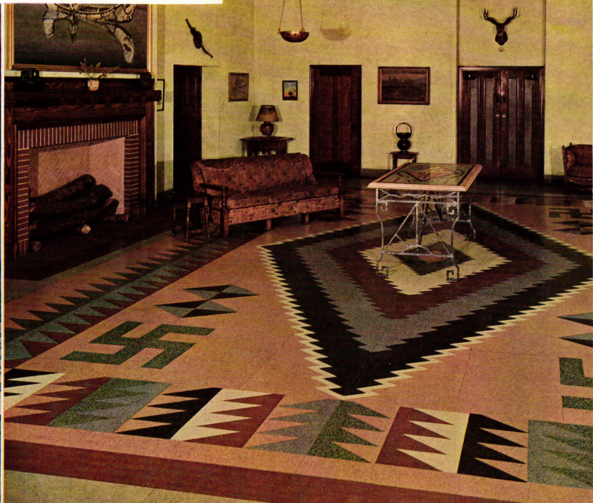
Indian rug design (below right) in FINE TERRAZZO made with Atlas White cement, in Friars Club, Cincinnati. Architects, Crowe & Schulte; Contractor, Martina Mosaic & Tile Company—both of Cincinnati.
