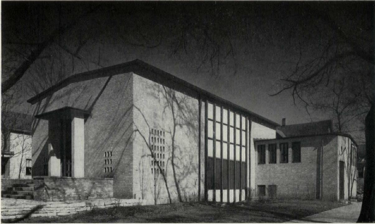
COMMON BRICK AND PRE-CAST CONCRETE ARE THE MATERIALS USED FOR THIS SIMPLE CHURCH
