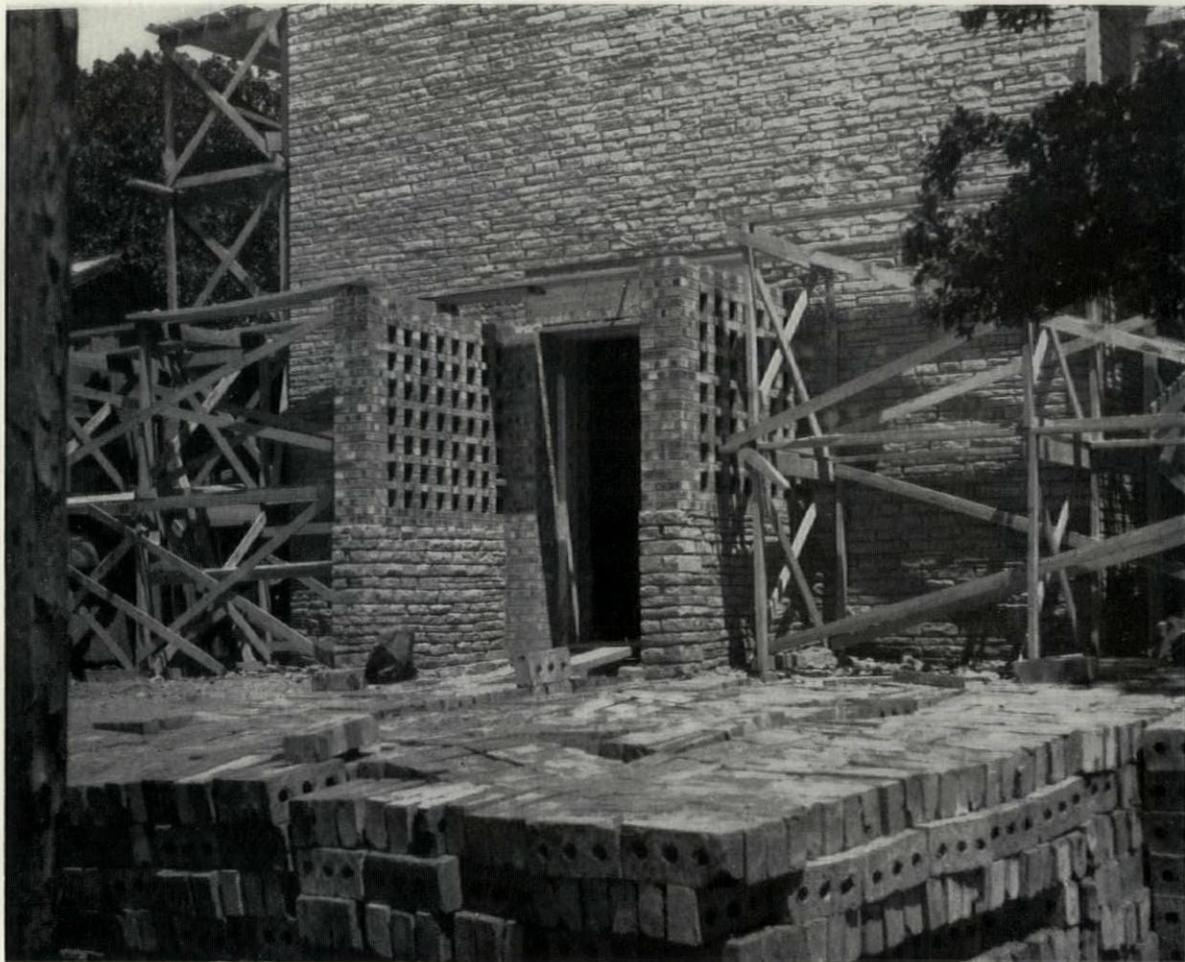
BRICK GRILLES ADD TO THE INTEREST OF THE CHAPEL ENTRANCE SHOWN, ABOVE, DURING CONSTRUCTION AND, AT RIGHT, AS COMPLETED. THE PORCH OPENS ON A VESTIBULE, OF WHICH THE WALLS ARE DECORATED WITH MOSAICS AND THE FLOOR MADE OF TEXAS STONE OF VARIOUS COLORS. PHOTOS FURNISHED BY THE NYA
