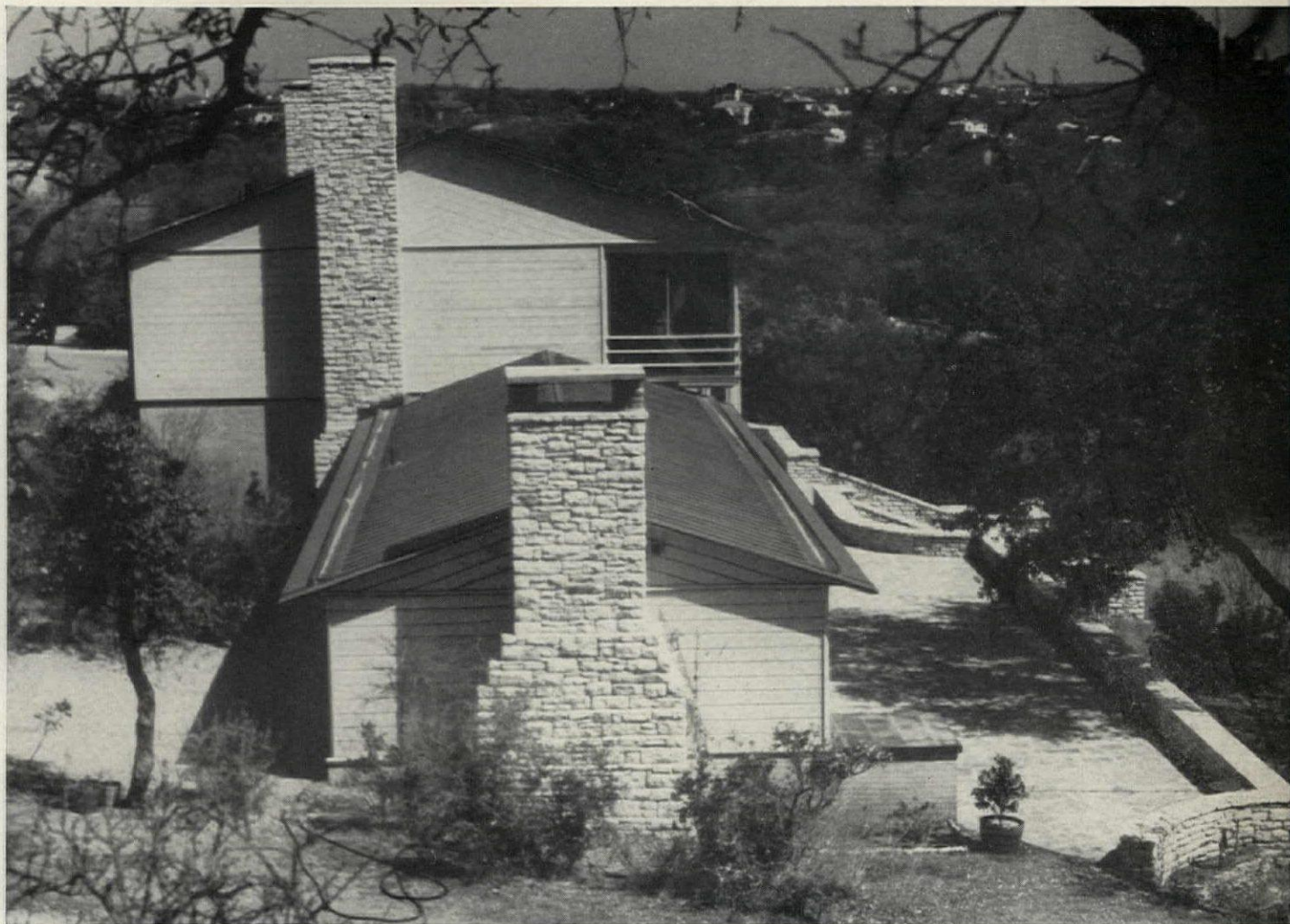
THE T. F. MURCHISON HOUSE ON A SLOPE ABOVE SAN ANTONIO HAS WIDE PORCHES AND MANY WINDOWS ON THE SOUTHEAST SIDE TO WELCOME THE PREVAILING BREEZES, BUT THE BLANK WALLS SEEN ABOVE SHUT OUT THE HOT AFTERNOON SUN ON THE SOUTHWEST SIDE. STONE FOR THE CHIMNEYS AND TERRACE WAS QUARRIED ON THE SITE, AND THE HOUSE IS SET COMFORTABLY IN THE NATIVE GROWTH
