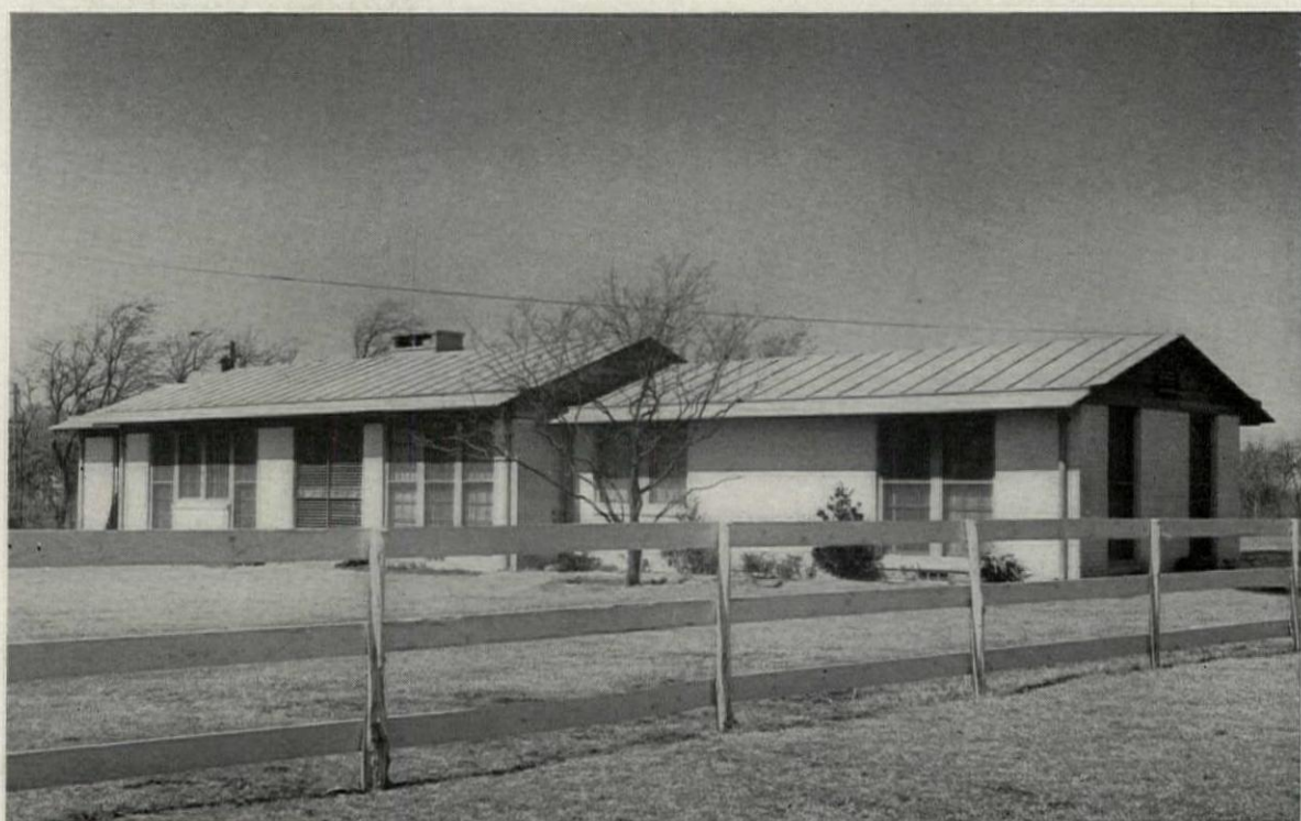
THIS VIEW OF THE HERSH HOUSE SHOWS THE SIMPLICITY OF THE FRAME STRUCTURE, ERECTED ON A REINFORCED CONCRETE SLAB. IT IS DEFINED BY ZISMAN AS THE "FIRST REAL TEXAS HOUSE OF THE PRESENT MOMENT." THE JOHN S. MAXSON HOUSE IN DALLAS (BELOW) HUGS THE FLAT PRAIRIE. WALLS ARE OF PAINTED BRICK, WITH NATURAL REDWOOD TRIM, AND WELL-INSULATED RIDGED METAL ROOF
